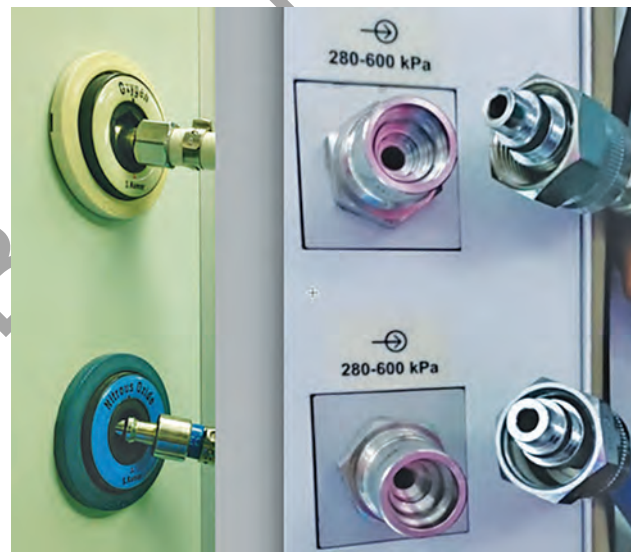
Fig. 2.8: Quick coupler on the left. Diameter index safety system connectors on right.
